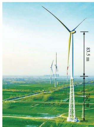
Fig. 1 Photo of the new tower and its surroundings
